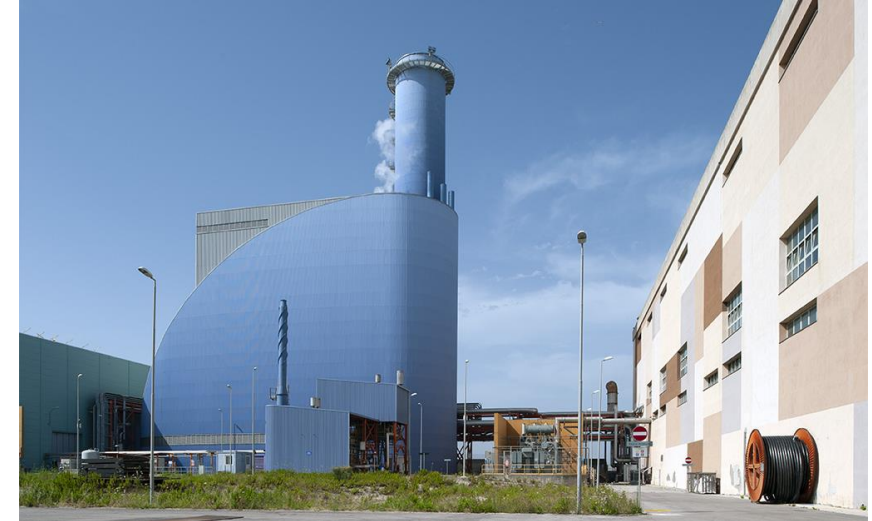
Napoli Levante power plant
