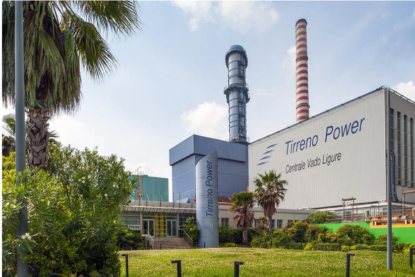
Centrale Vado Ligure power plant
